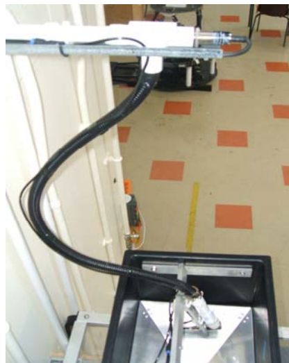
Figure 3-17 Use of Flexible Conduit
