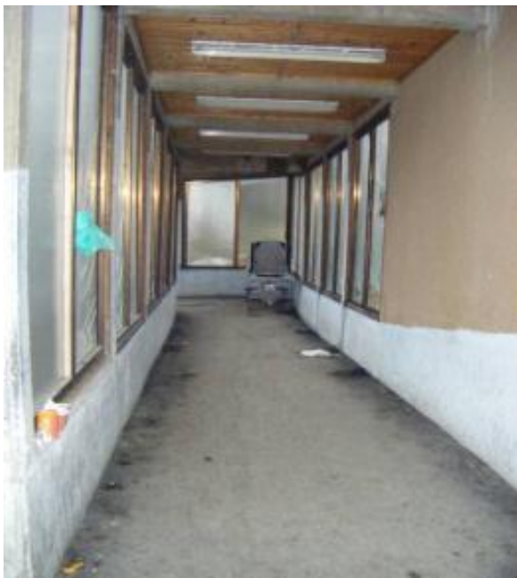
Figure 6 Top of the Ramp
