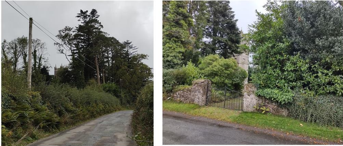
Figure 7.8: View of the Church of Ireland chapel from two directions on the road, partially hidden by the low walls, tall trees and vegetation
